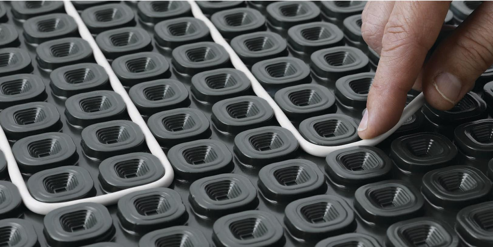
Warm Tiles® Electric Floor Warming Cable for Uncoupling Membrane is the easy-to-install, reliable solution for your floor warming project.
