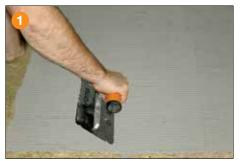
Using a thin-set mortar that is suitable for the substrate, apply the thin-set mortar (mixed to a fairly fluid consistency, but still able to hold a notch) using a  $1/4" \times 3/16"$  (6 mm x 5 mm) V-notched trowel,  $5/16" \times 5/16"$  (8 mm x 8 mm) V-notched trowel, or the DITRA trowel, which features a  $11/64" \times 11/64"$  (4.5 mm x 4.5 mm) square-notched design.
