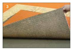
Lift up a corner of the matting to check coverage. Proper installation results in full contact between the fleece webbing and the thin-set mortar. Simply abut end and side sections of adjacent sheets.
