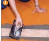
Comb additional unmodified thin-set mortar over the joint using a 1/4" x 3/16" (6 mm x 5 mm) V-notched trowel or the Schluter®-KERDI trowel, which features a 1/8" x 1/8" (3 mm x 3 mm) square-notched design. Using the flat side of the trowel, firmly press the 5" (127 mm)-wide Schluter®-KERDI-BAND into the mortar to ensure 100% coverage and to remove excess mortar and air pockets.
