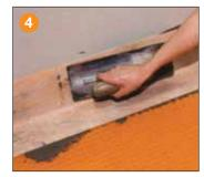
At all wall junctions, apply a 10" (254 mm)-wide strip of KERDI-BAND as described in steps 1-3, centered where the wall and floor meet.
