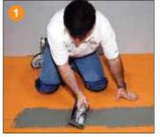
At the joints, fill the cut-back cavities with unmodified thin-set mortar, approximately 8" (203 mm) wide, centered over the joint.
