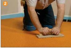
Apply DITRA or DITRA-XL to the floor, fleece side down. Solidly embed the matting into the bonding mortar using a float, screed trowel, or Schluter®-DITRA-ROLLER (please observe the open time of the bonding mortar).
